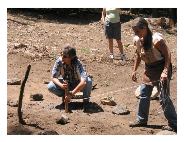
Now you're ready. Make a small loop in the end of your rope. Then make three knots, spaced about one arm length (yours) apart. Pound your stake into the ground just far enough to make it solid if you slightly tug on the rope. Put the loop around the stake so it can swivel freely as you walk around the circle.
